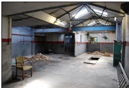
Ground Floor Internal No. 55
