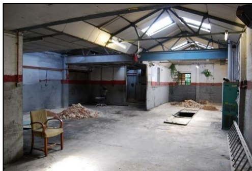
Ground Floor Internal No. 55
