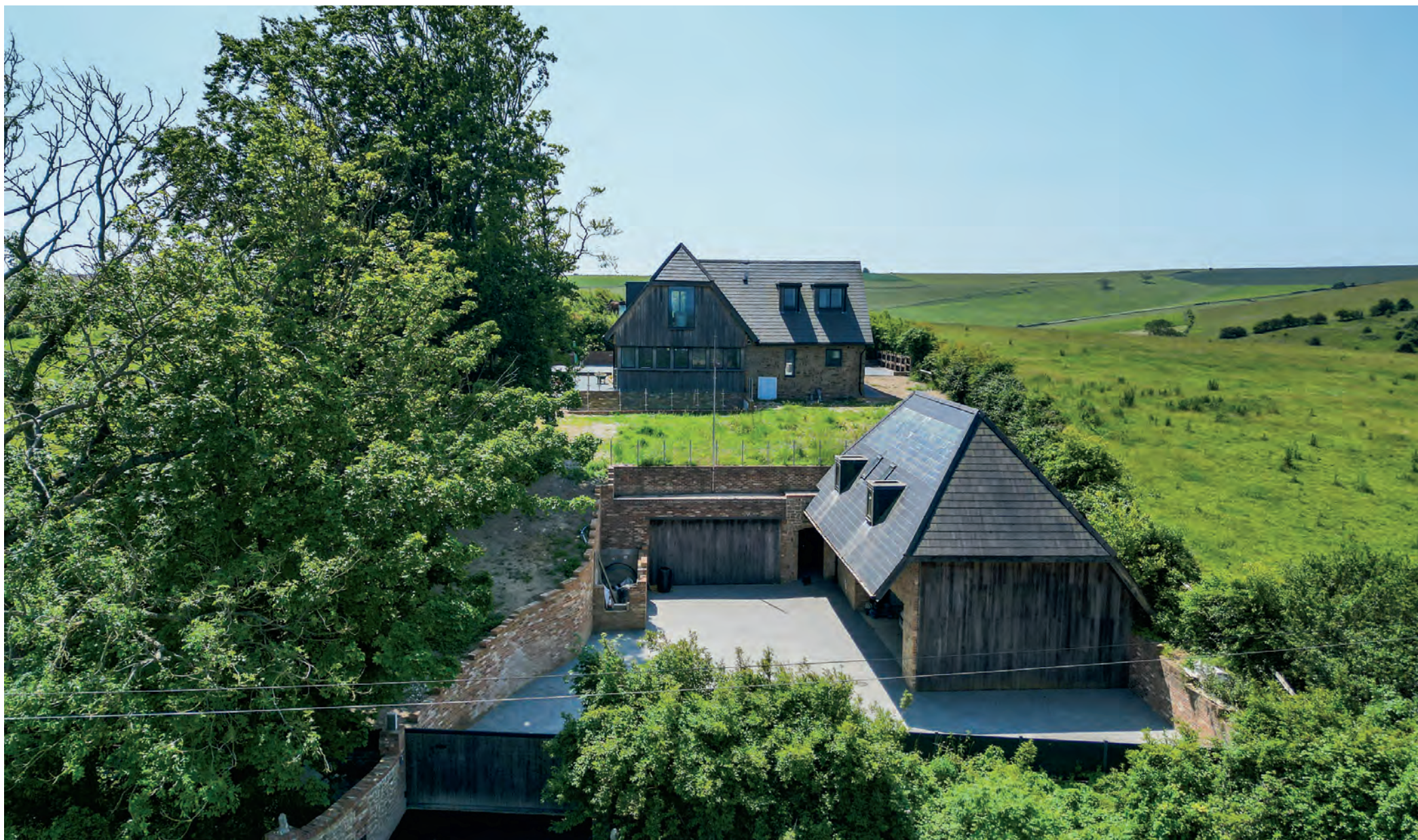
Highfields Cottage Bostal Road | Steyning | West Sussex | BN44 3PD
