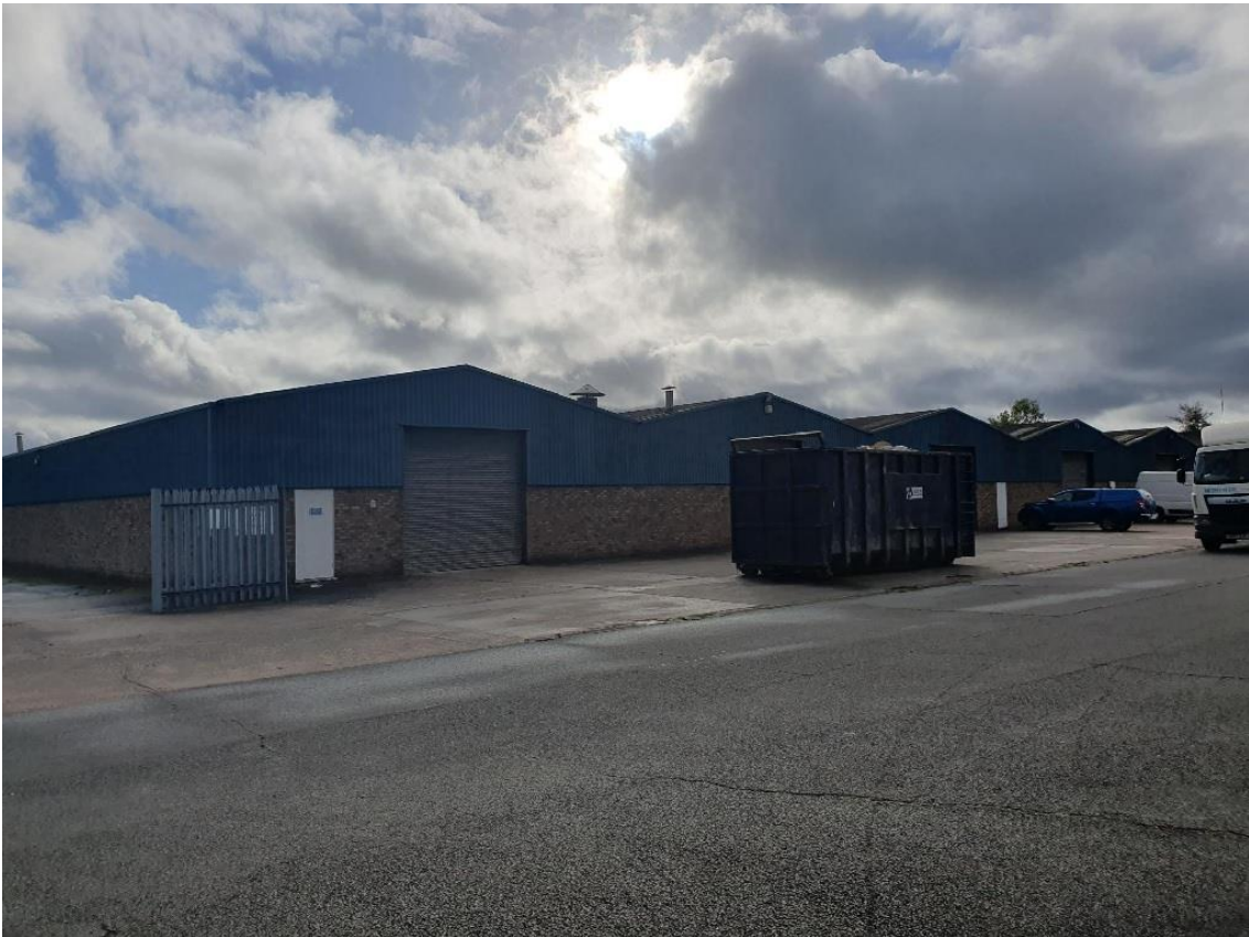
UNIT SHOWN PRE-REFURBISHMENT
