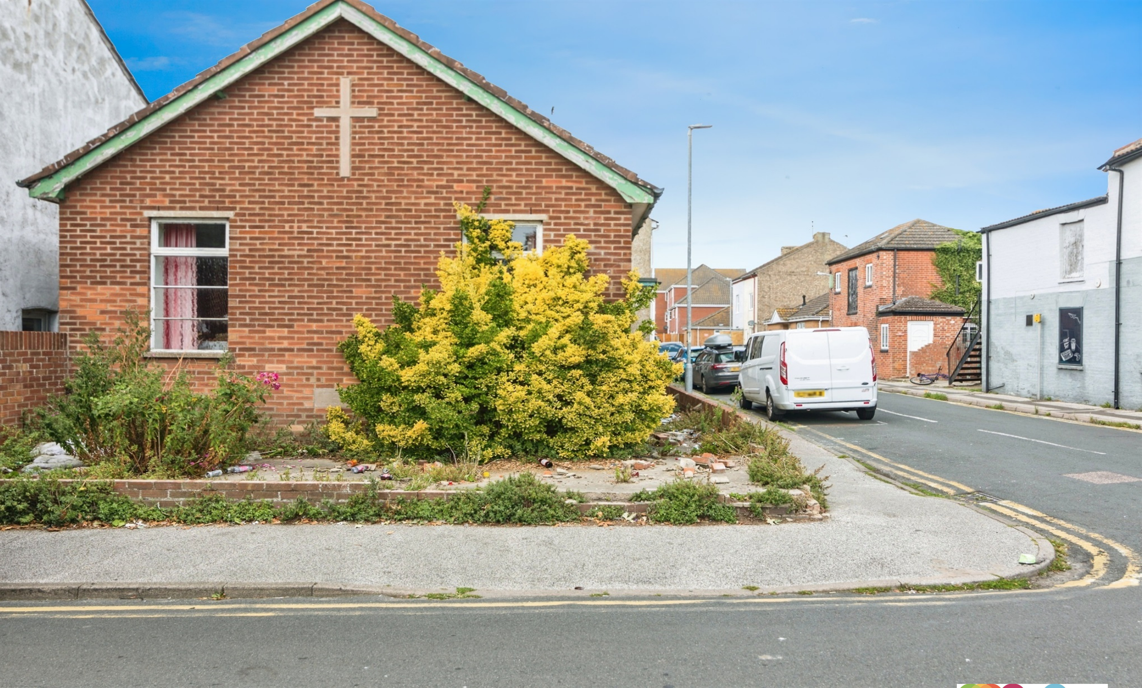
Lowestoft Wesleyan Reform Chapel Raglan Street, Lowestoft NR32 2JS
