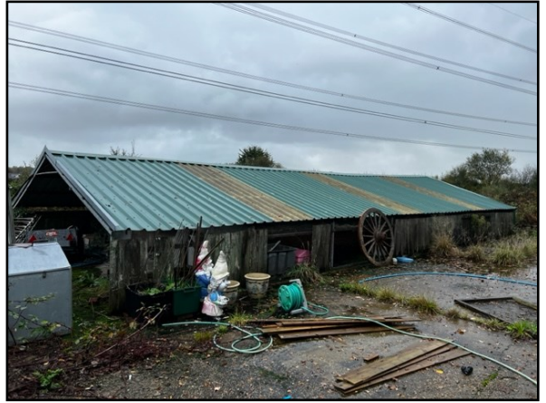
POULTRY BUILDING - LOT 3
