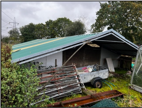
POULTRY BUILDING - LOT 3
