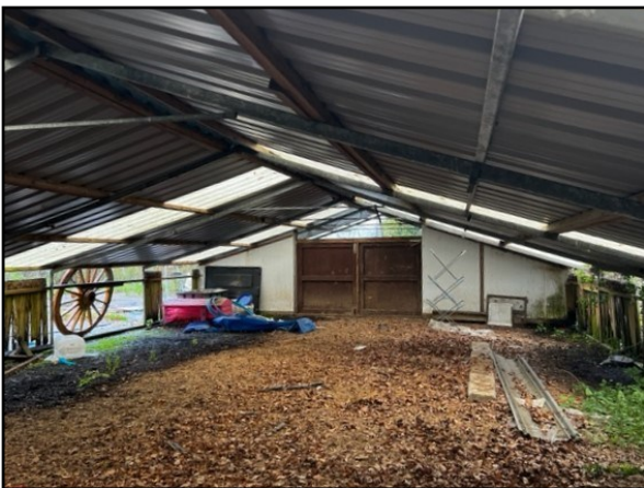
POULTRY BUILDING - LOT 3
