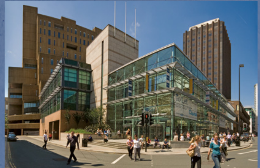
The Capital is the largest office building in Liverpool, at 410,000 sq ft. Formerly the HQ of Royal and Sun Alliance. Re-positioned as Grade A office space and let to The Borders Agency as their Regional Consolidation hub.
