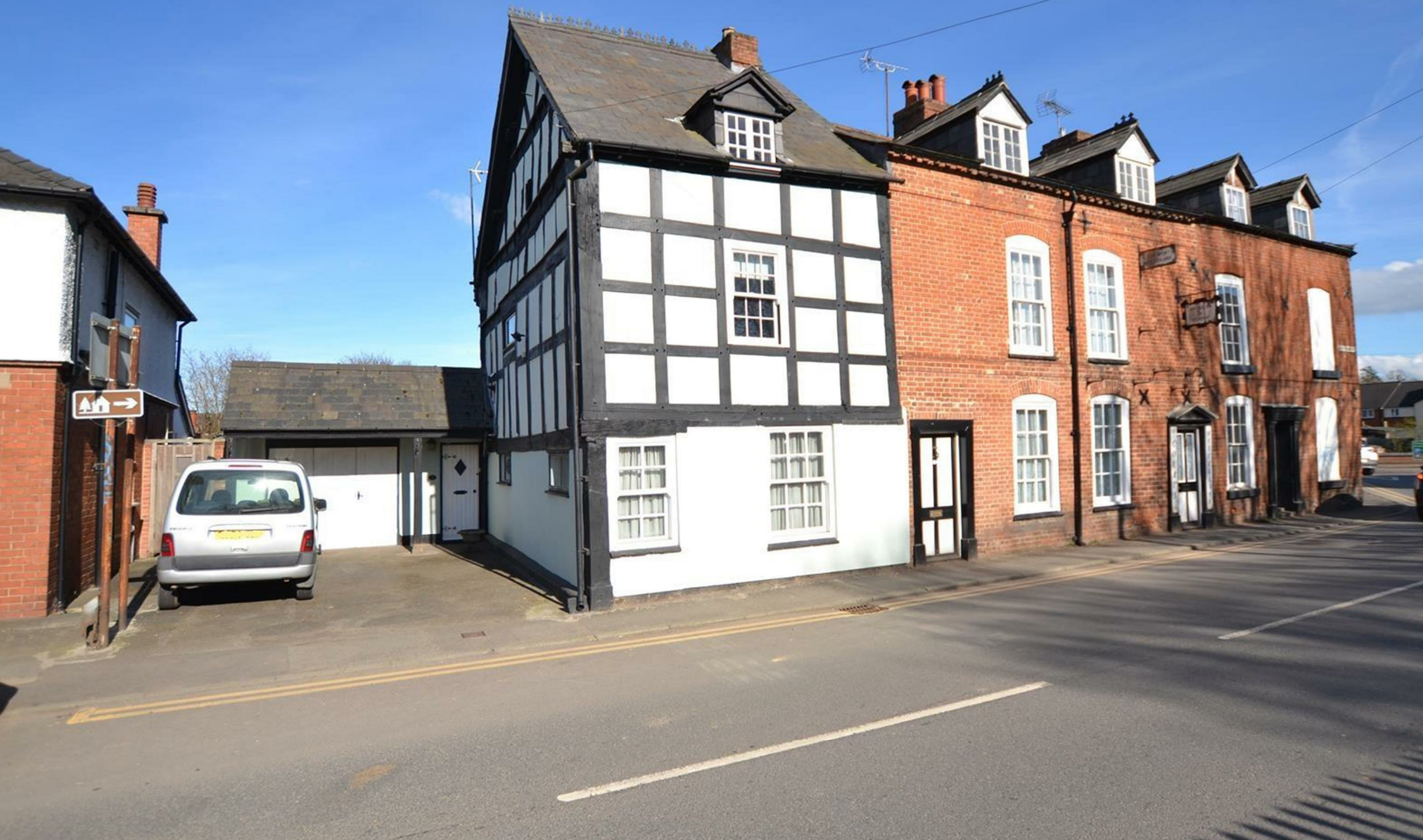
52 Bridge Street, Leominster, HR6 8DZ. £260,000
