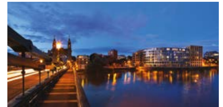
QUEENS WHARF, W6 165 residences right on the banks of the Thames adjacent to Grade II listed Hammersmith Bridge. A joint venture with Mount Anvil.
