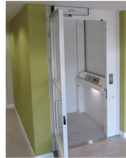
Easy Access to lower ground, ground and first floor via full mobility lift
