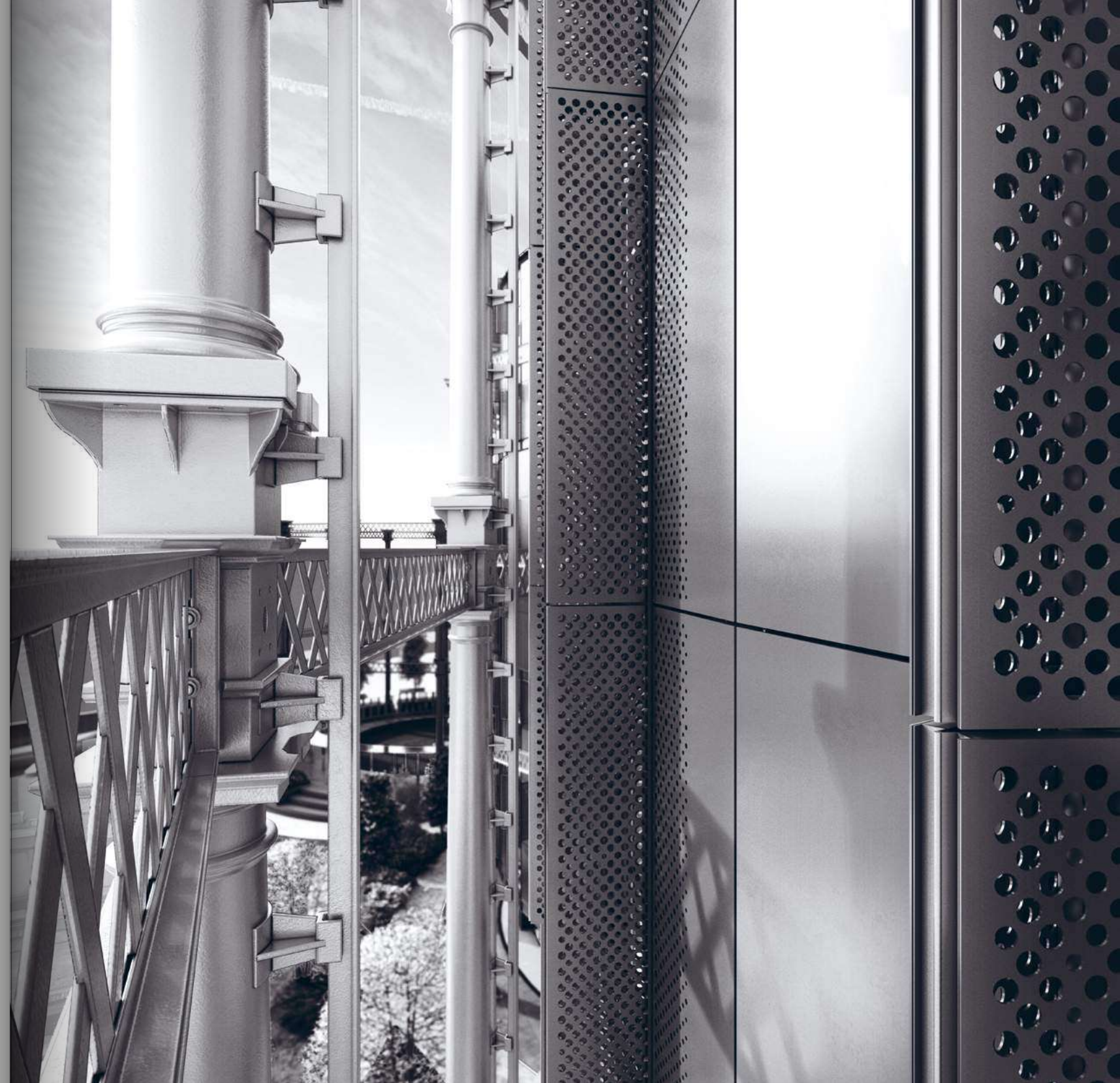
The façade of flickering contemporary metals and neighbouring Victorian frames, with views looking out over London
