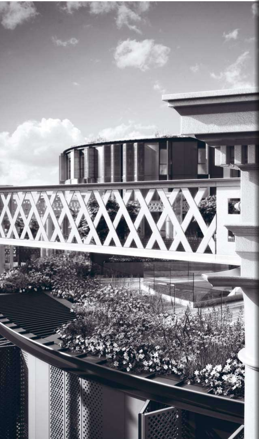
Gasholder 12 has a residents' roof garden designed by landscape design practice Dan Pearson Studio
