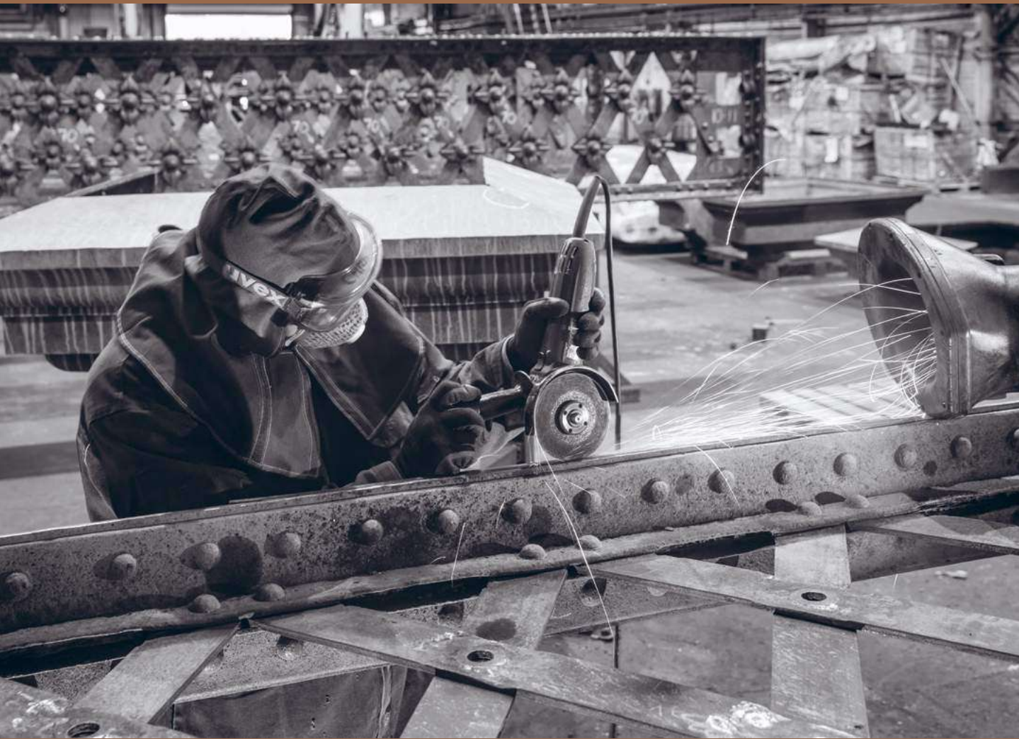
It has taken over two years to painstakingly refurbish the 123 cast-iron gasholders columns
