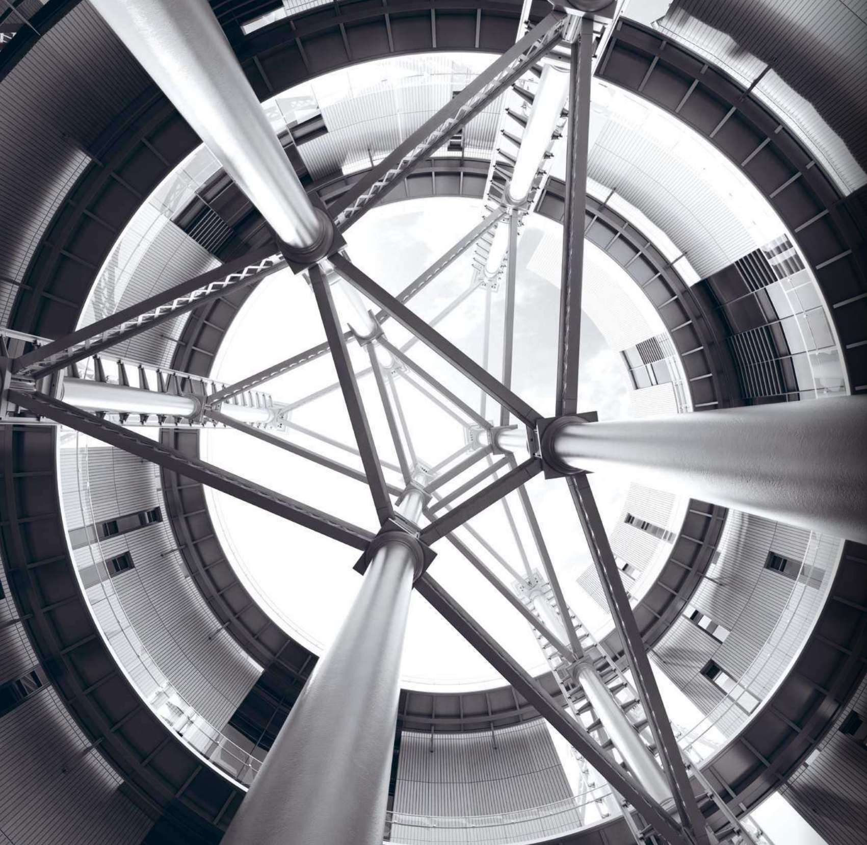
Looking skywards through the structure from within the central courtyard
