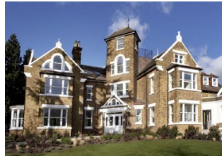
Theydon Towers, Epping
