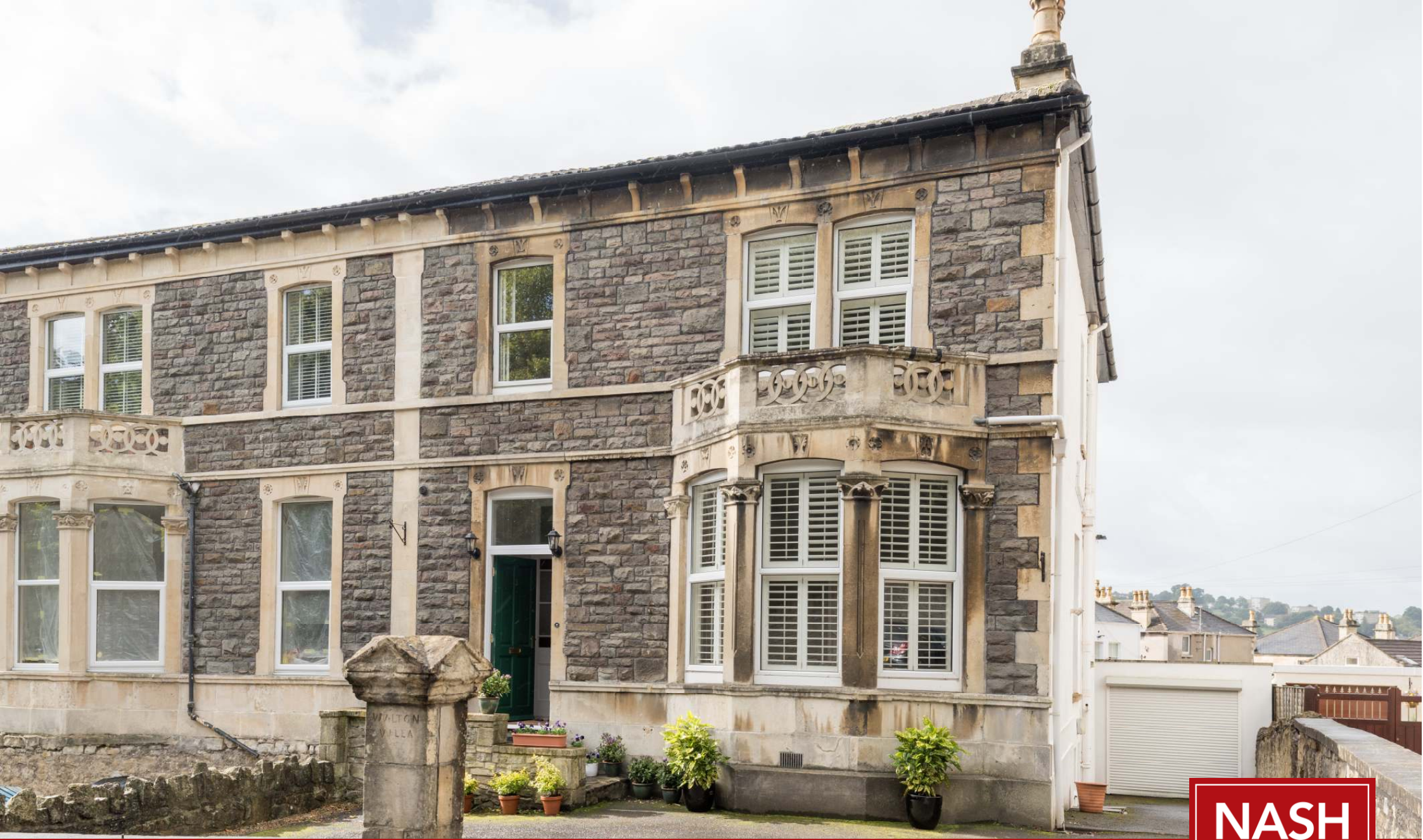
Newbridge Hill Newbridge | Bath
