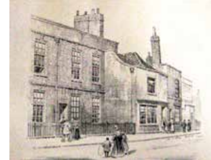
Original hospital building
