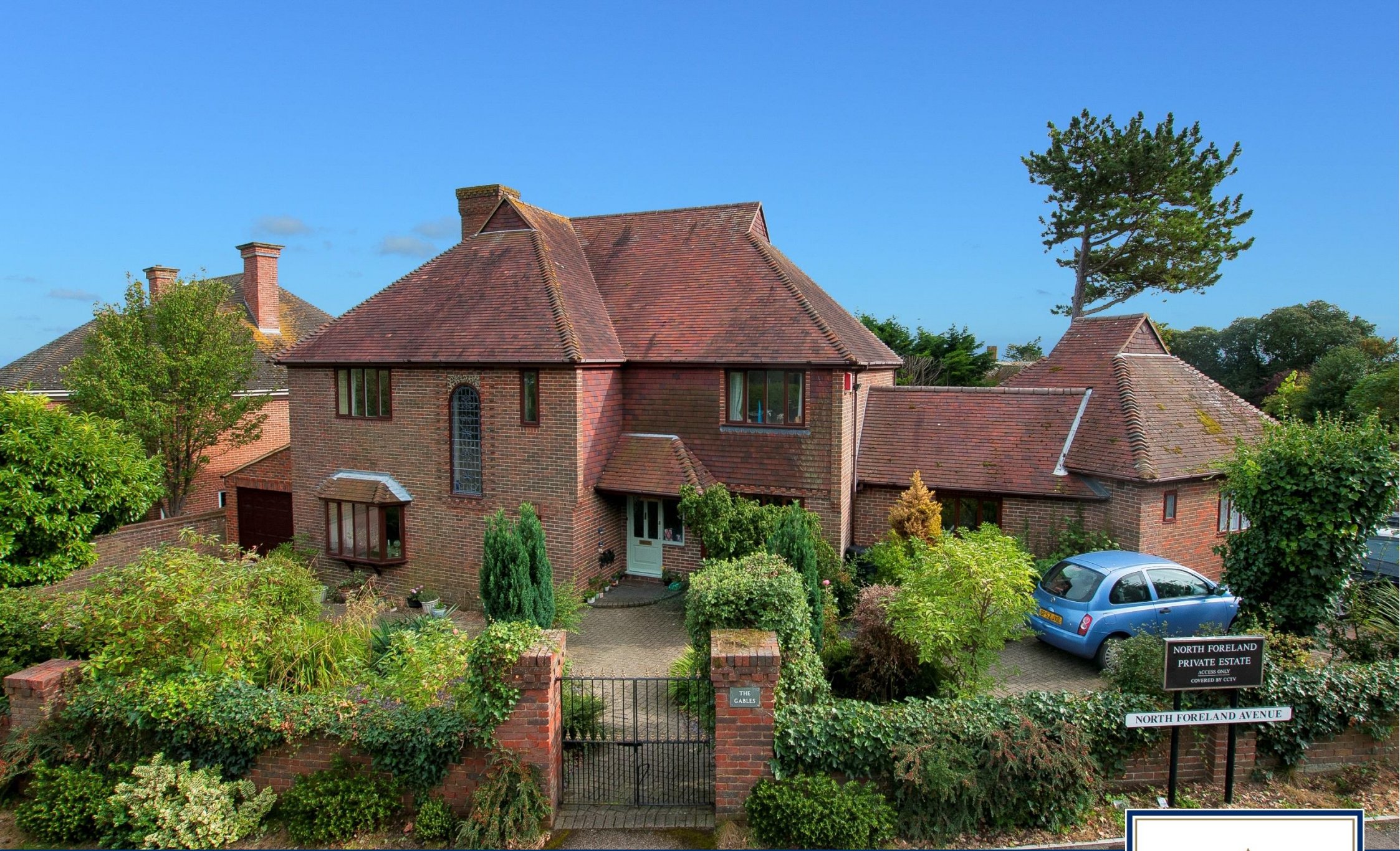
North Foreland Avenue, Broadstairs
